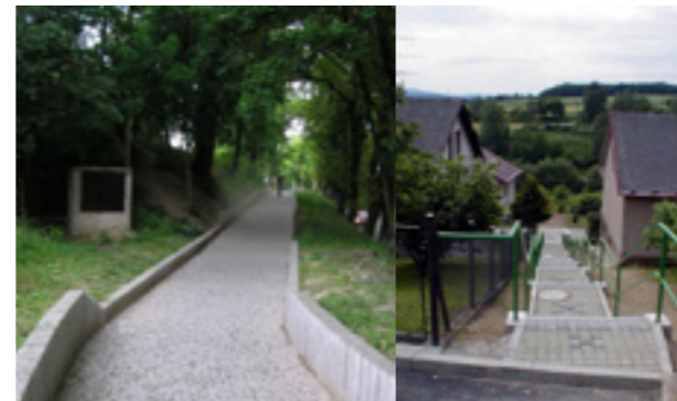
2.23 - 2.24 Paving Ensure comfortable walking in rainy weather.
