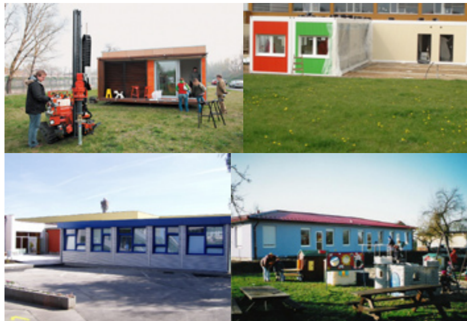
2.14 - 2.17 Modular structures Examples of fast assembled and easy to remove modular structures used for school buildings. (exhibition example, Dolní Břežany, Prague, Kimmer - Germany)
