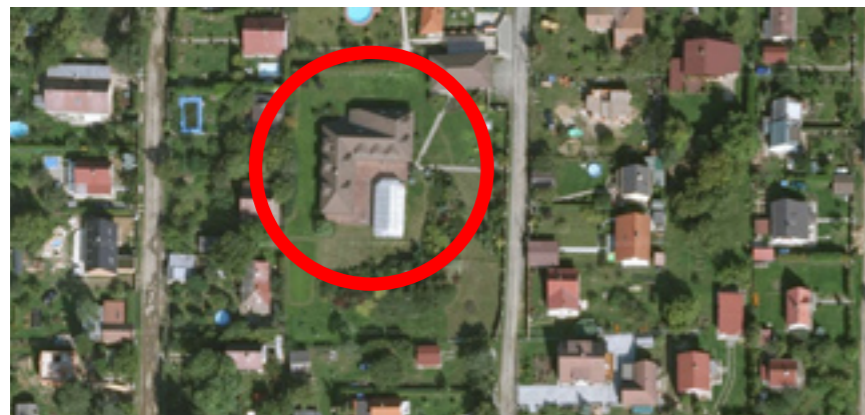
2.18 Unplanned transformation New building in the weekend house colony not respecting the scale and character of the place. (Zálepy)
